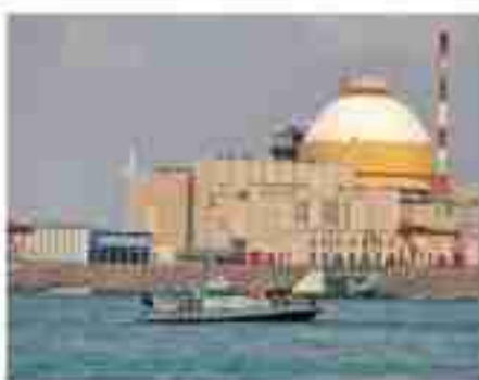
Nuclear reform: Currently, only three PSUs can build and operate nuclear power plants in the country, it is noted
